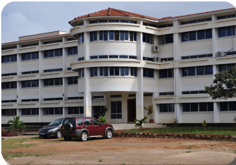
The New Administration Block
