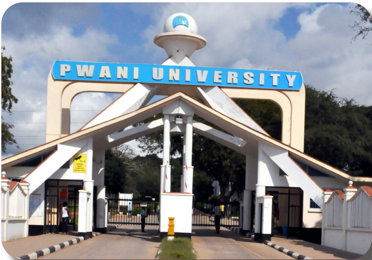
The New Main gate
