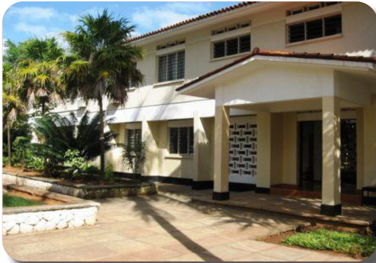
The Old Administration Block
